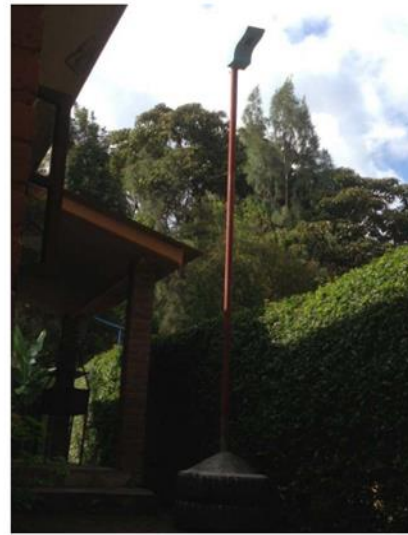
Mounted on concrete-filled old tire with greased pole in Tanzania
